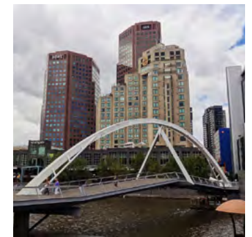
Top: William Barak Bridge. Above: River Yarra (Rainbow) Pedestrian Bridge.
