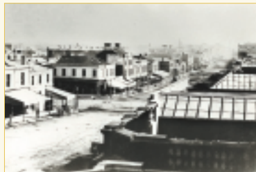
Swanston Street circa 1849 from St. Paul's Church under construction.
